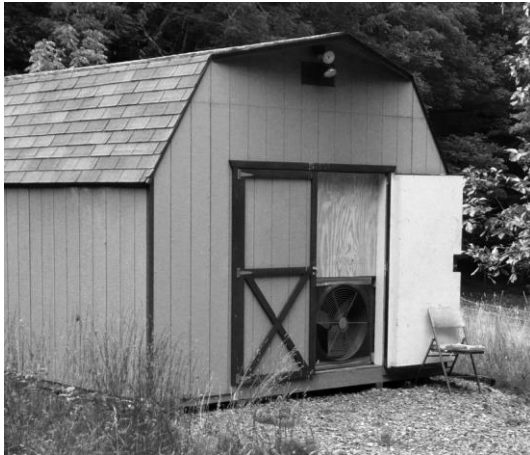
Figure 3. Inside this shed used for apple storage is Big Bucks Pit, a 43 m. drop into Barberry Cave. The pit is sealed to the floor of the building. The door to the building has been reduced to the size of the fan. Accordingly, as the fan blows in and out of the building the air is exchanged in the cave.
